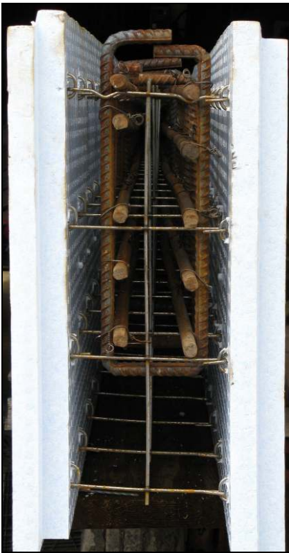
Picture 2.5.a - Reinforcement structure for multi storey institutional project
