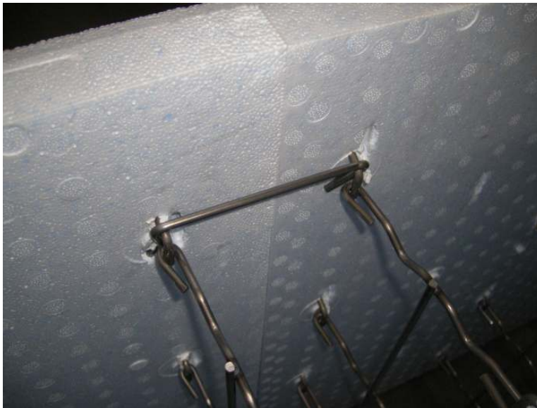
Image 2.1.3.b – Joint bracket installation
